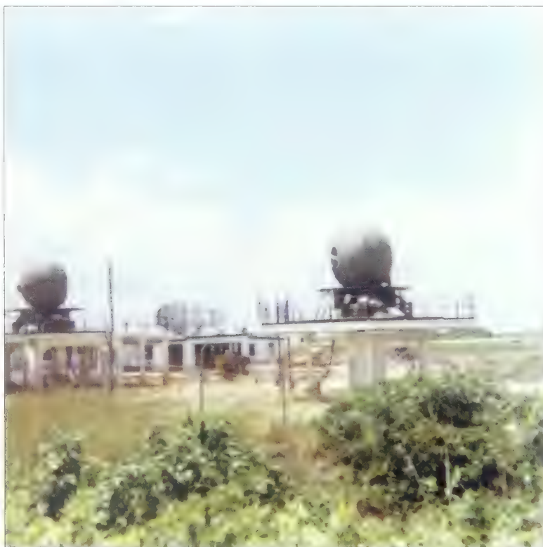
Figure 5.103. View looking west at target tracking radars (417 and 473), Control Area #1, NIKE radar site, circa 1962. The vegetation in the foreground of this image was located in front of the perimeter fence and was outside the site. Beyond the fence and around the radar platforms was bare sand, beachgrass, and no woody vegetation (GATE 22043).
